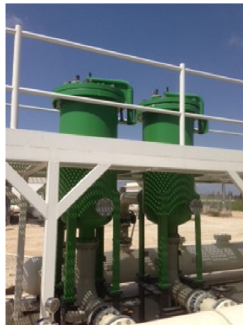
Cage design brackish water filter suitable for 400 m 3 /h flow-rate equipped with no. 80 x L 50" cartridges.
