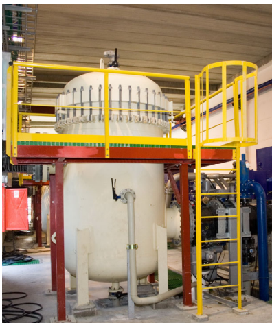
Cage design sea water filter suitable for 2000 m 3 /h flow-rate equipped with no. 400 x L 50" cartridges.
